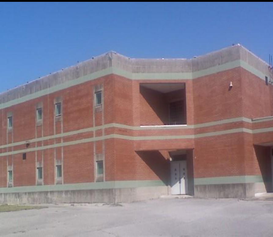
Moton Elementary School built in the early 1980's
